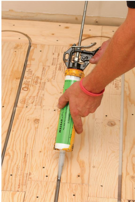
**Figure 26:** Apply a thin,  $\frac{1}{8}$ " bead of 100% silicone sealant to the entire length of the Quik Trak straight panel grooves. Do not apply the silicone sealant to the return panel grooves.
