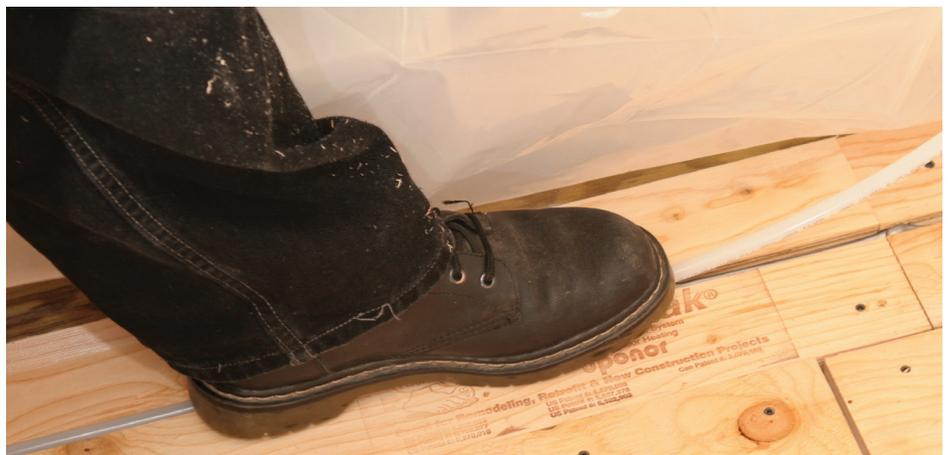
**Figure 27:** Use hard-soled boots or shoes to walk the piping into the panel groove.
