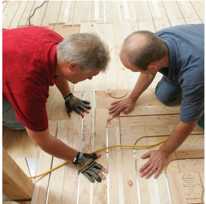
**Figure 3: Installing Quik Trak straight panels**
