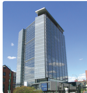
Manitoba Hydro Place, Winnipeg, Man. LEED Platinum
