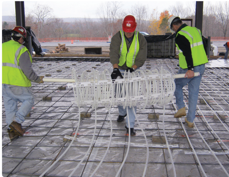
Figure 4-21: Uponor Radiant Rollout Mats are delivered to the job site in 5-foot or 10-foot wide sections that are rolled out onto the prepared grade, significantly reducing installation time and labor.
